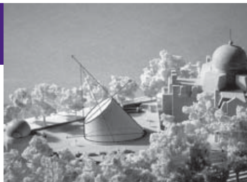
A model of the new 120-seat planetarium at the Royal Observatory. The building is in the shape of a truncated cone, angled at the latitude of Greenwich, 51.5°.
